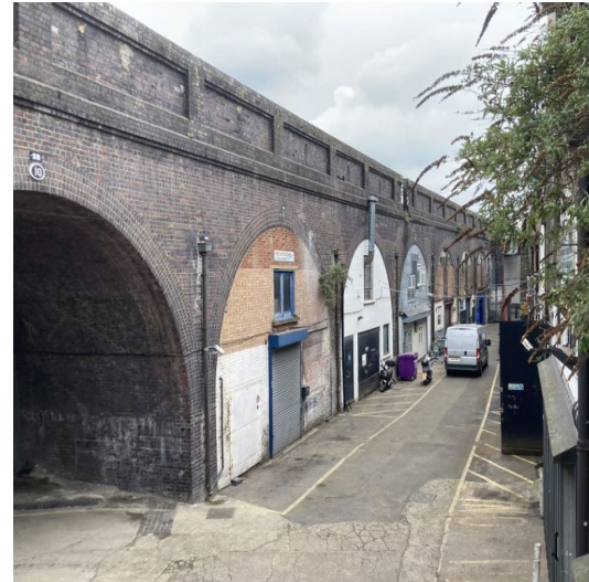
Kilburn Arches (Phase 1 - Mews)
