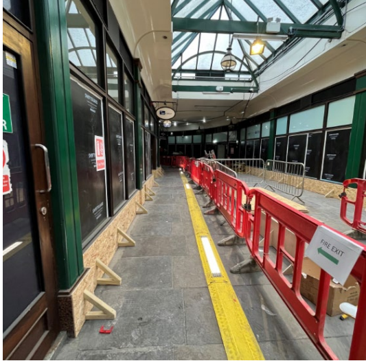
Liverpool Street Arcade
